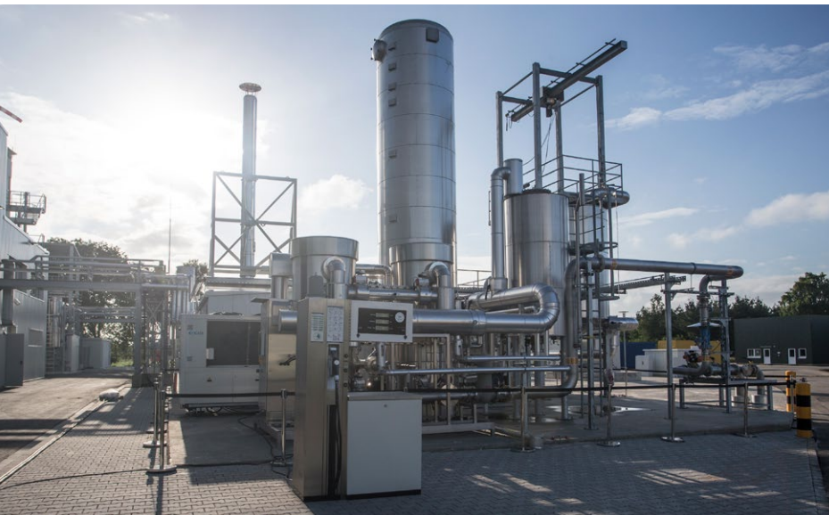
HZIBM amine scrubbing is a component of the power-to-gas plant in Werlte, Germany (Photo: Audi AG)
